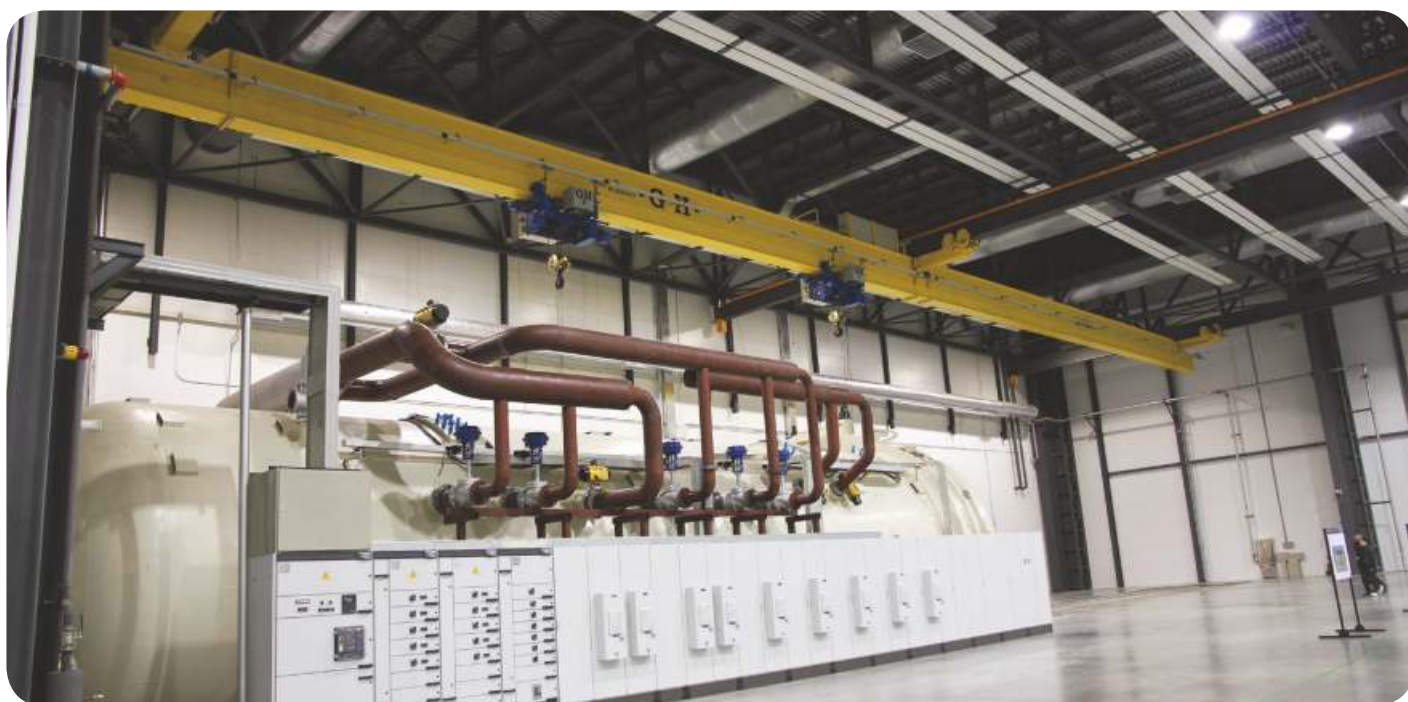
MULTIPOINT SINGLE GIRDER UNDERSLUNG CRANE. CAPACITY UP TO 20+20t. 多支点单梁悬挂起重机，额定载荷达20+20吨
