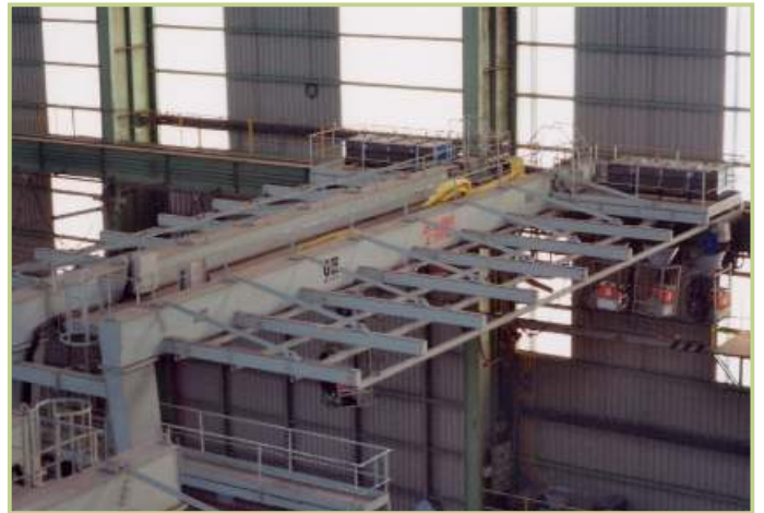
■ SUPPORT STRUCTURE FOR WELDING EQUIPMENT
